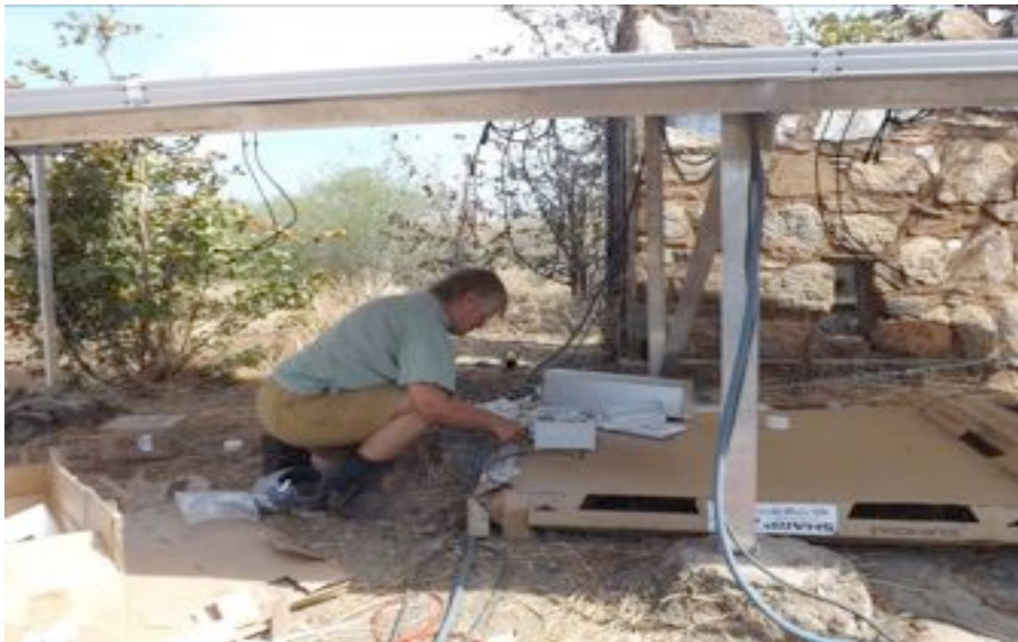
Connecting the electrics
