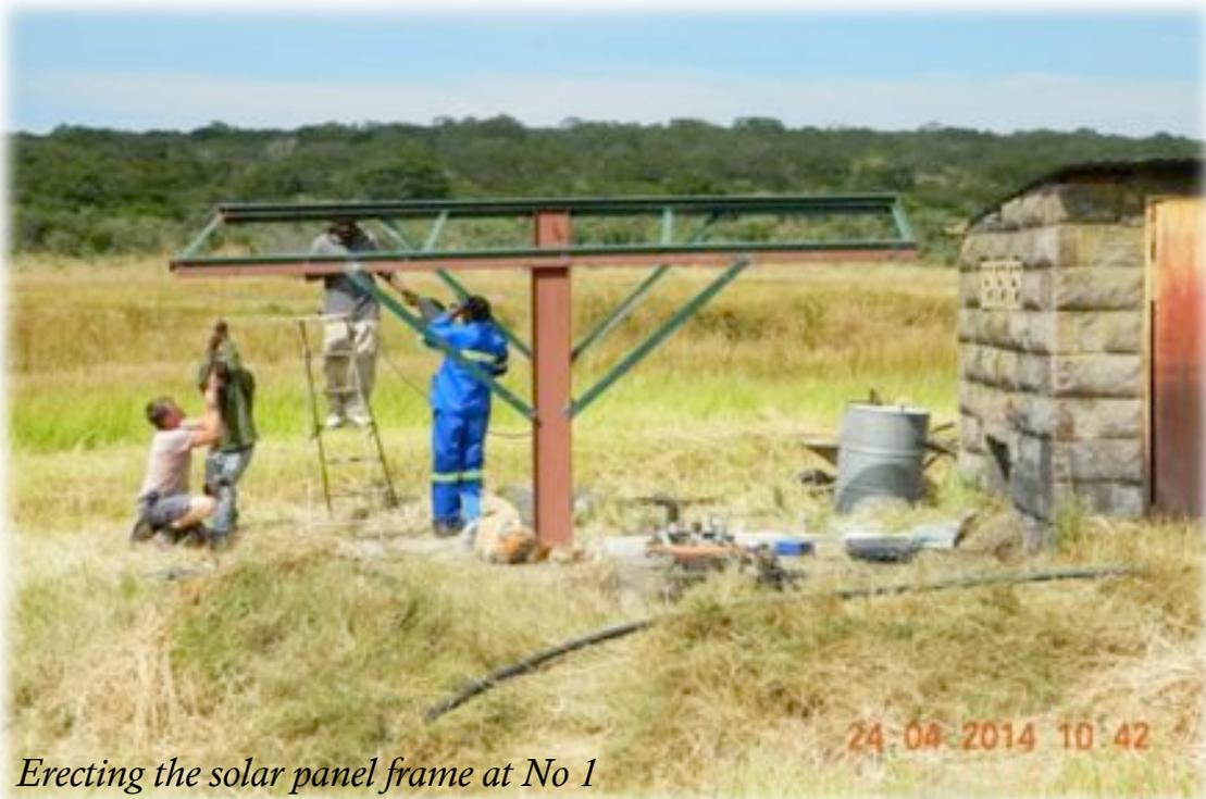
*Erecting the solar panel frame at No 1*
