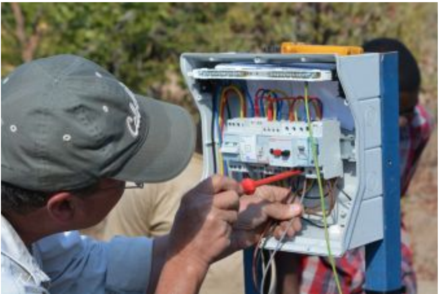
Dave connecting the pump wiring to the switchbox – No 5
